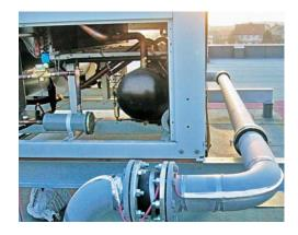
Silicon elastomer Insulation
